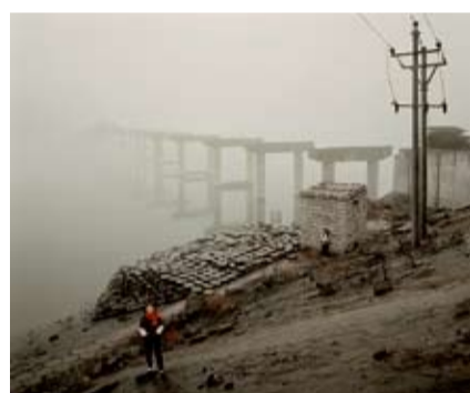
萬州·斷橋 Broken bridge in Wanzhou
