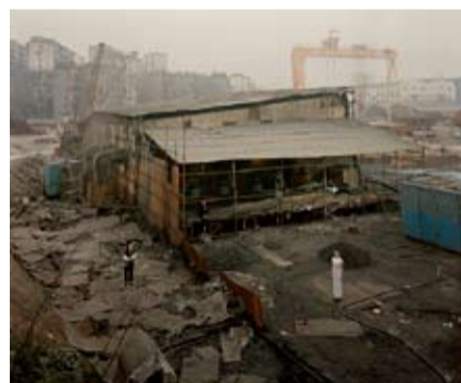
重慶·噴漆車間 A garage in Chongqing
