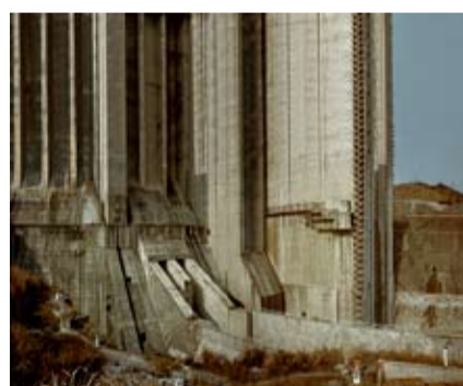
宜昌·三峽大壩 The Three Gorges Dam, Yichang
