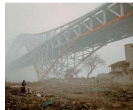
重慶·長江新橋 New bridge on Yangtze River, Chongqing
