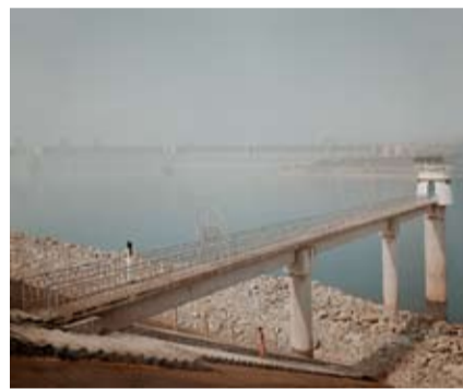
宜昌·三峽水文站 Three Gorges Monitoring Station, Yichang
