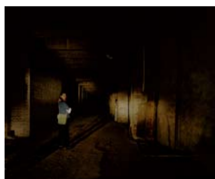
涪陵·28公裏長的核工廠 Nuclear Plant stretching 28 km in Fuling
