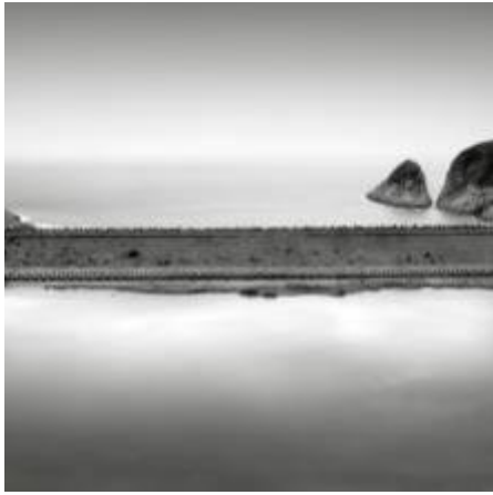
High Island Reservoir Dam, Hong Kong – 2008, Photograph
